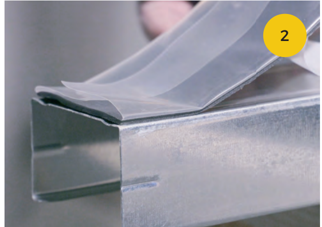
2. Place the sealing tape with the adhesive side centred onto C / U section
