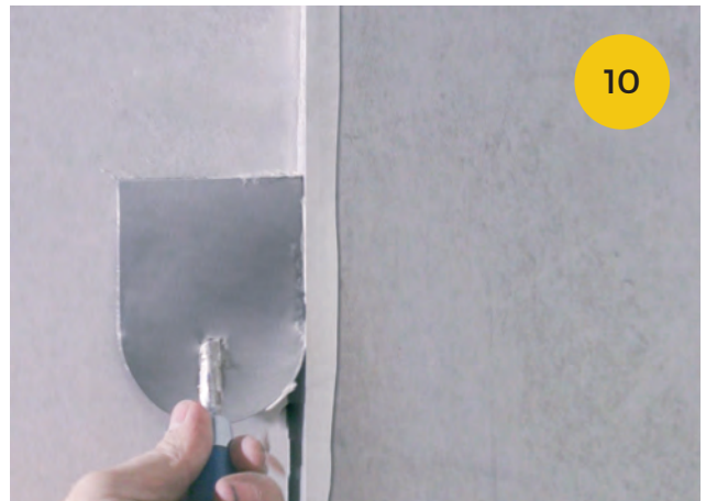
10. Fill the joints professionally
