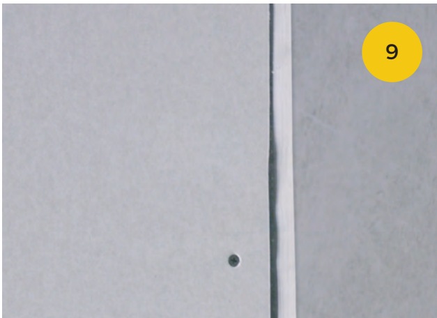
9. Mount the gypsum / fibreboard with at least 3-5 mm gap to the Montape® divider strips
