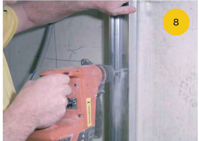
8. Fix the C / U section
