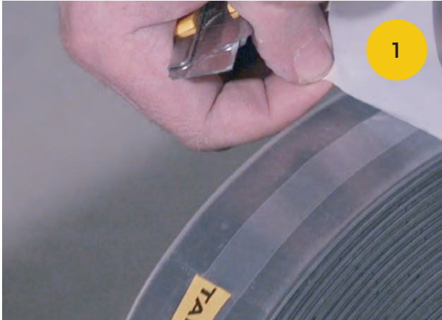
1. Peel off the silicone foil from the underside of Montape®
