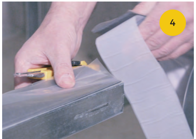
4. Cut off Montape®
